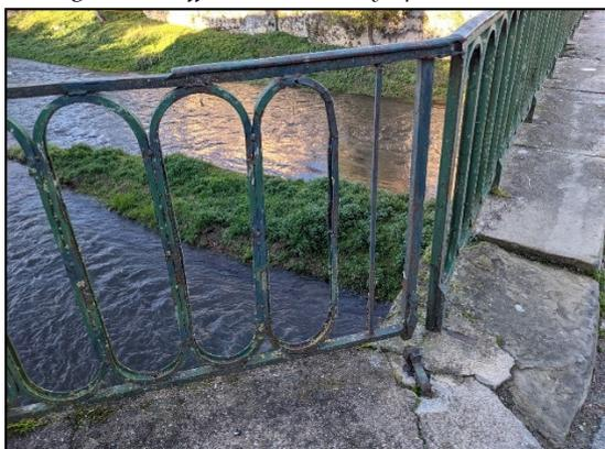
*Figure 12 : Montant garde-corps cisailé*
